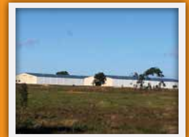
Machinery Sheds - Bundaberg, Qld
