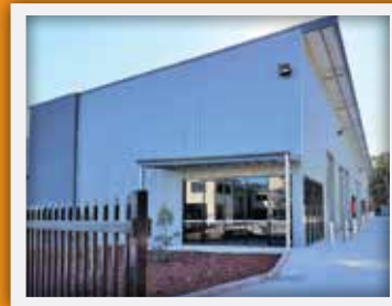
Industrial Units – Bennetts Green, NSW
