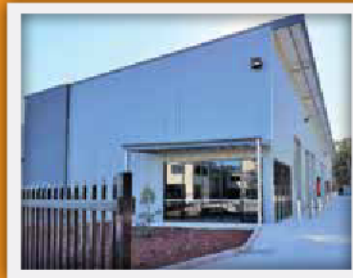
Industrial Units – Bennetts Green, NSW
