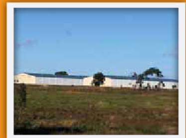
Machinery Sheds - Bundaberg, Qld
